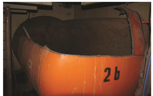
Storage tank during segmentation
