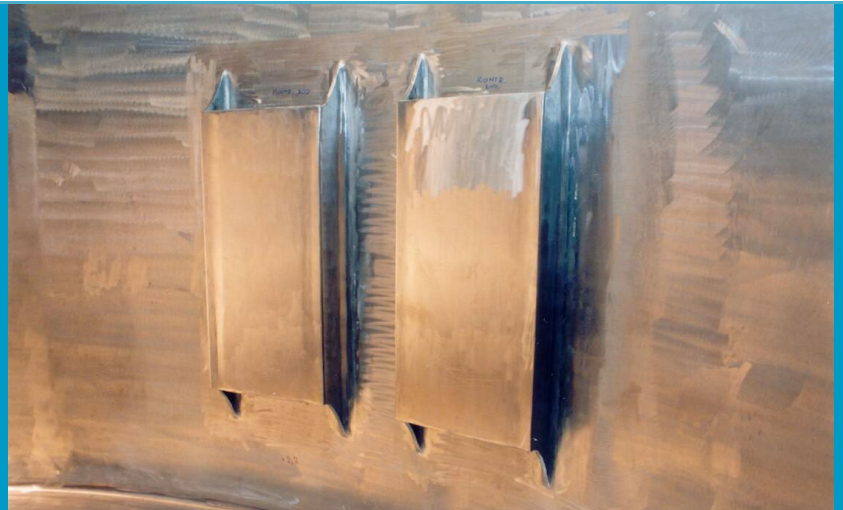
Reactor pressure vessel inner wall capsule holder for VVER-1000 (Temelin NPP)
