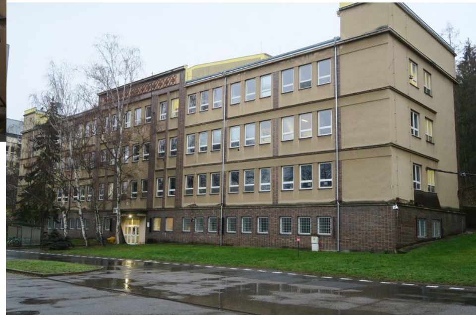
Reactor building administrative and operation part
