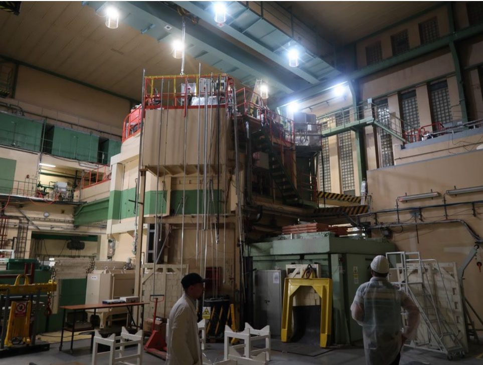
Heavy concrete reactor shaft in reactor hall
