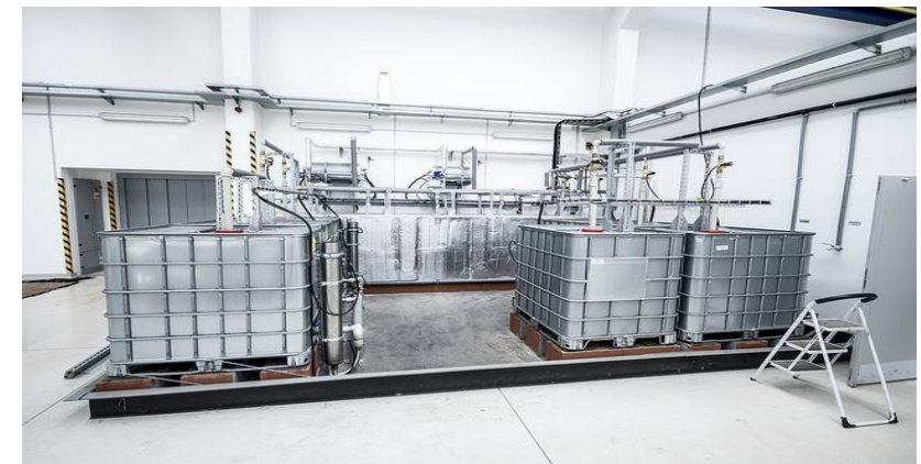
Spray solution system
