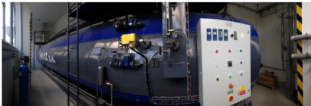
Steam boiler for generating steam
