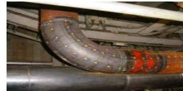
Flow accelerated corrosion
