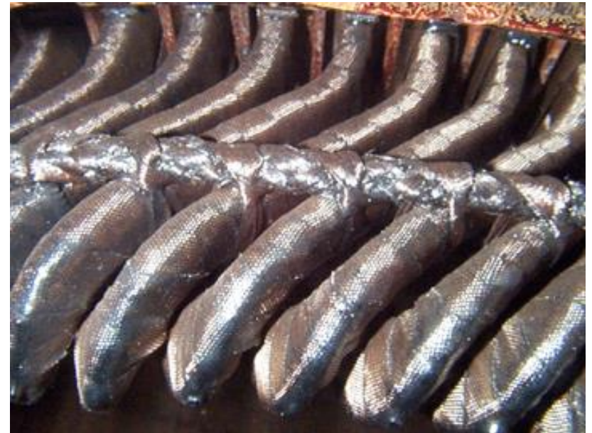
Surge ring material and ties on the opposite connection end
