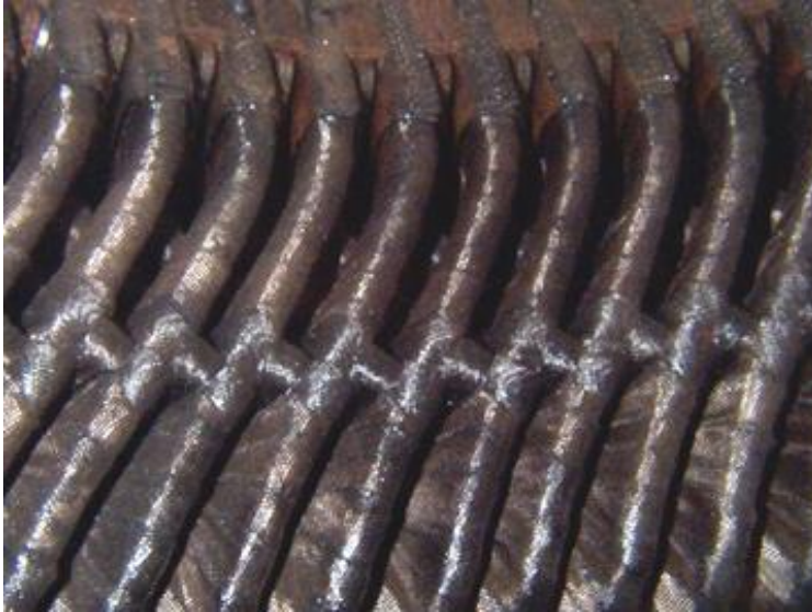
Opposite connection end “butterfly” tying/bracing.
