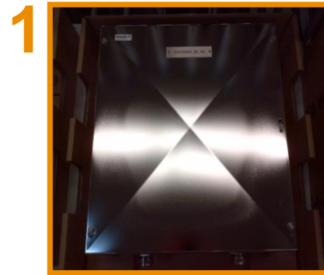
Reinforcement of the lid
